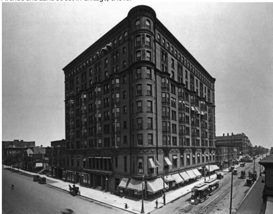
The Lexington Hotel, located at the corner of Michigan Avenue and 22nd Street in Chicago, c.1910.
