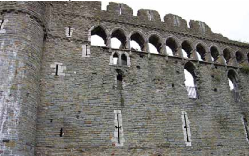
Arcading on south external wall.
